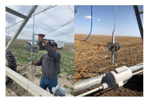
Step 6: With the cable in place, the manifolds with leader lines of Dragon Flex hose should now be unrolled and attached to the cable. Hang the manifolds to the cable loosely with wire or other device to allow for easier handling. Using the wire ties provided manifold should be tied to the cable at each tee and each adaptor tee used to feed water to manifold. Wire ties should wrap around the cable at least two to
