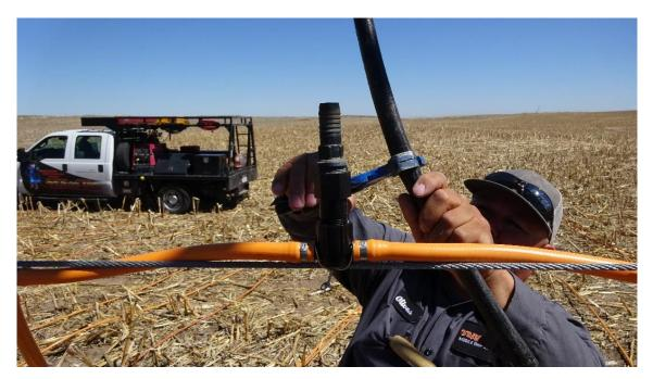
Step 8: Using nozzle chart provided, cut Dragon-Lines to length according to drop number and end plug can then be installed at the end of the drip line. For easier install (especially in colder weather) drip lines can be cut and end plugs can be installed in a shop to then be taken to the field. This makes install take less total time as measuring.
